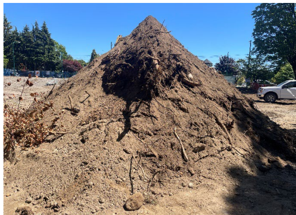
Figure 6 Excavated material removed via dump truck
