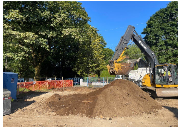
Figure 5 Physical removal via excavator
