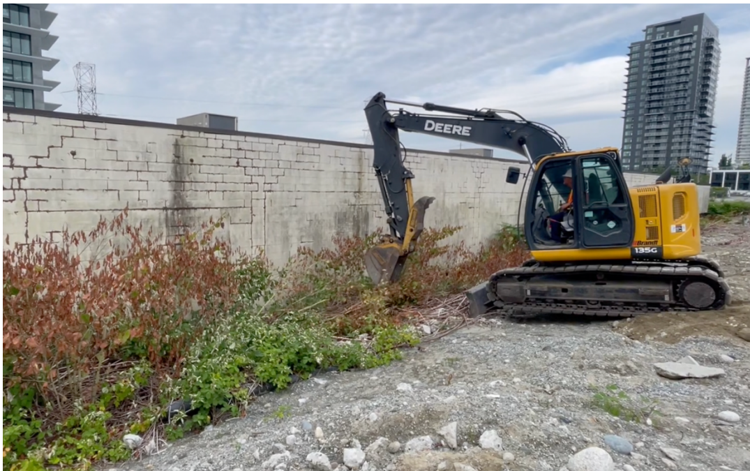
Figure 4: Excavation up to 3 meters underground
